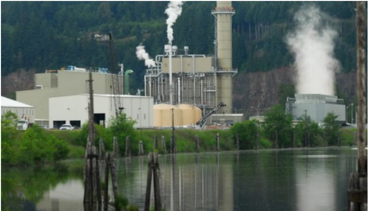
PGE's Port Westward gas-fired power plant near Clatskanie.
