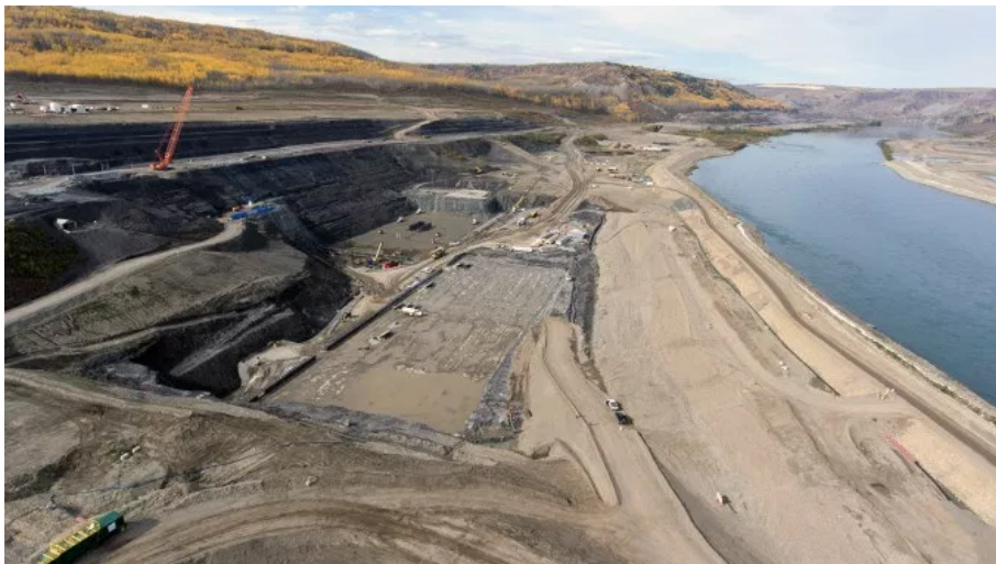
An aerial view of the south bank excavation at Site C, including the stilling basin and the powerhouse buttress, in September 2017. Photo by BC Hydro
