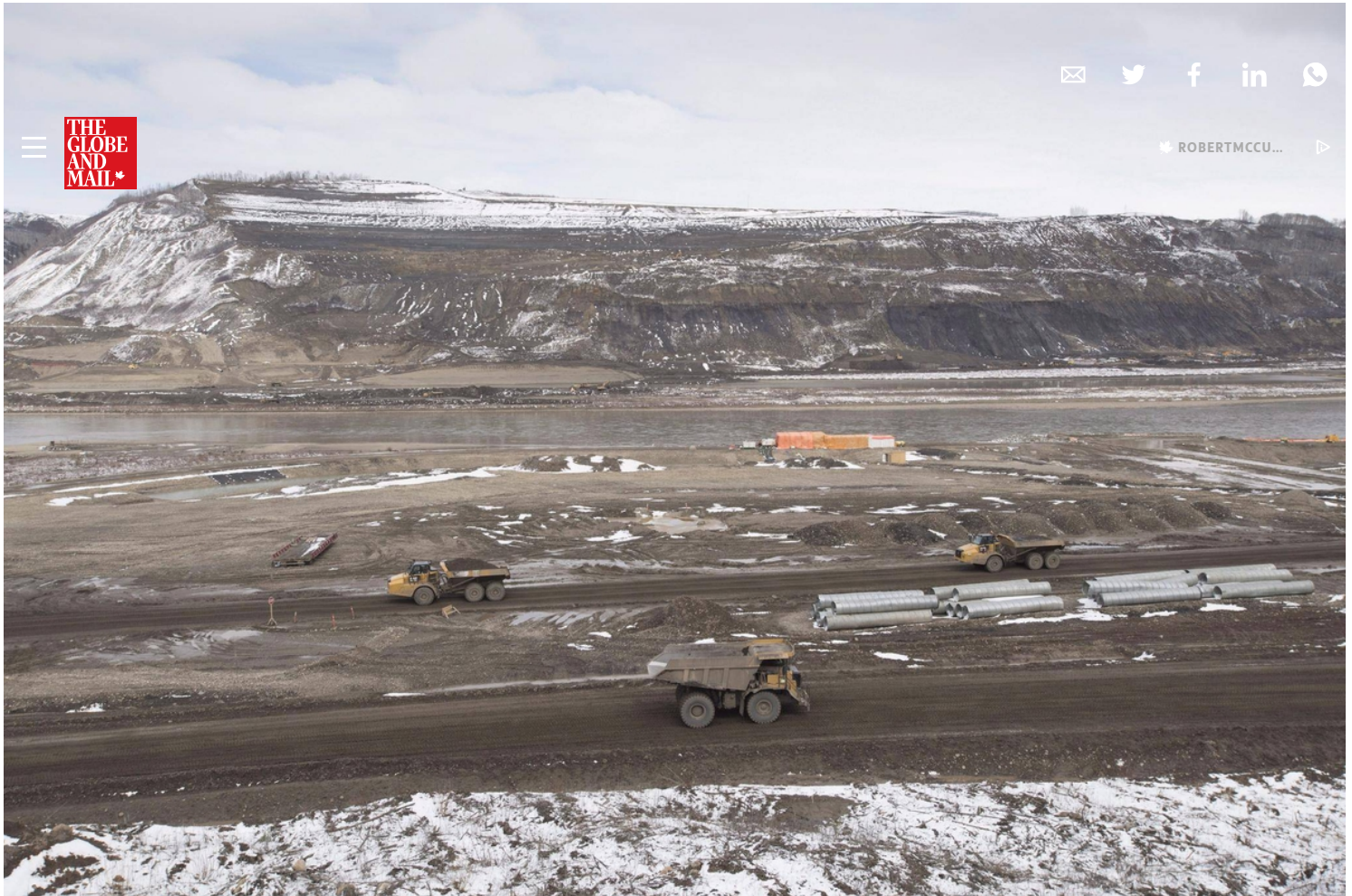
The Site C Dam location is seen along the Peace River in Fort St. John, B.C., Tuesday, April 18, 2017.
