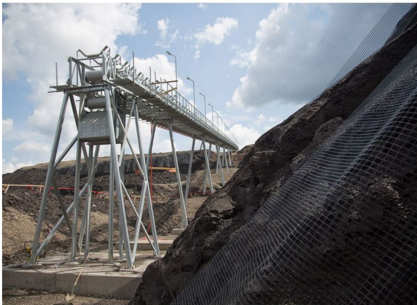
Roller-compacted, concrete-conveyor construction at the south bank of B.C. Hydro's Site C dam project near Fort St. John. B.C. HYDRO
