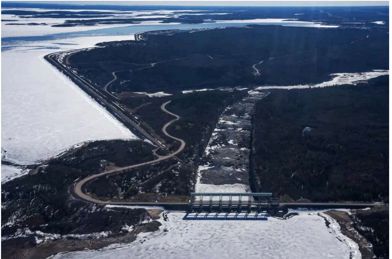
The Robert-Bourassa hydroelectric dam and its spillway, along La Grande River.
