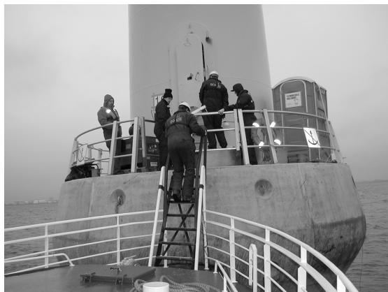
Figure 6: A safe access to the foundation is essential when the waves and current are moving the ship.
