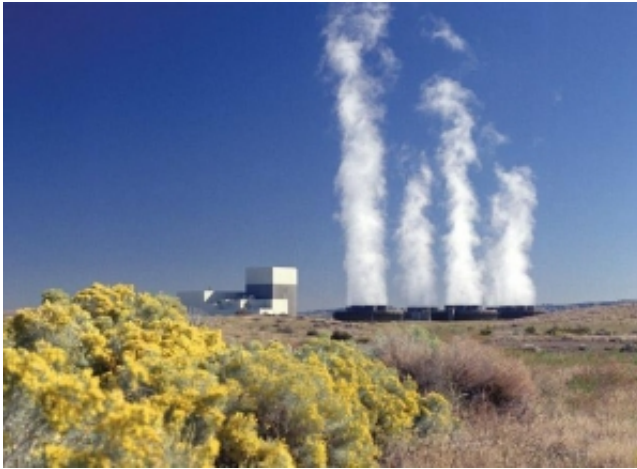
Energy Northwest's Nuclear Plant in Richland, Wash. - Energy Northwest
