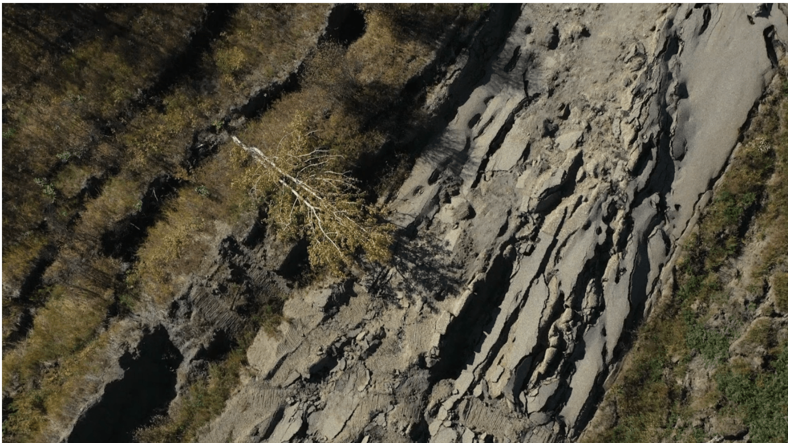
The Old Fort road, crumpled by a November 2018 landslide on the notoriously unstable slopes of the Peace River. Photo: Jayce Hawkins / The Narwhal
